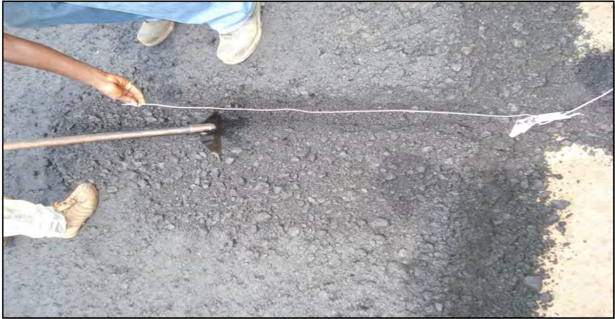
Figure 4.21 - Installation of thermocouple Sensor in Asphaltic concrete layer
