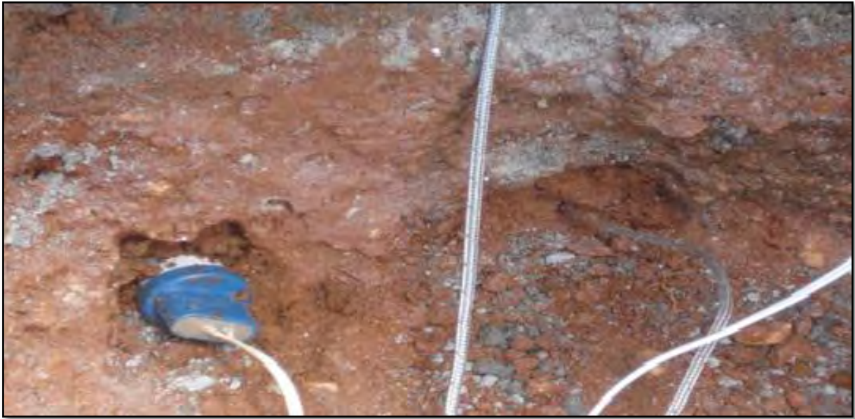
Figure 4.22 – Installed Moisture Block
