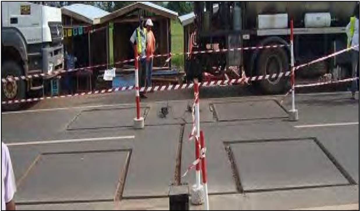
Figure 4.6 – Field Construction of Induction Loops Site
