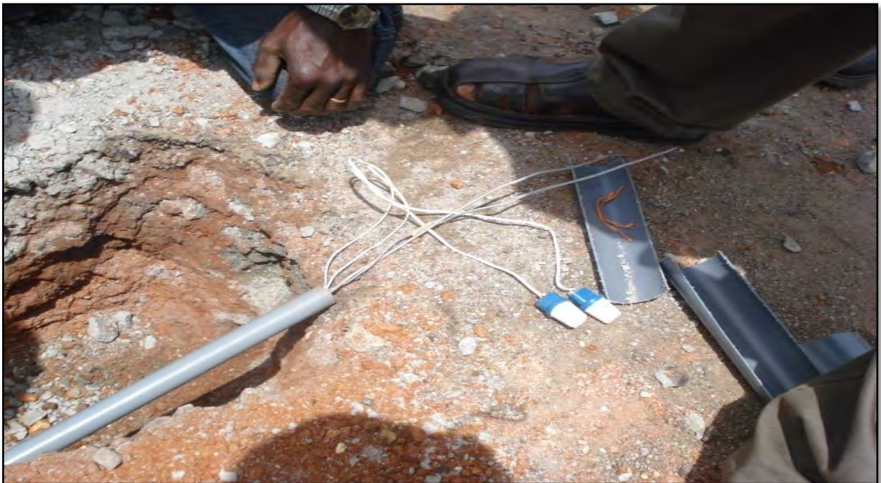
Figure 4.18 – Field Installation of Moisture Blocks
