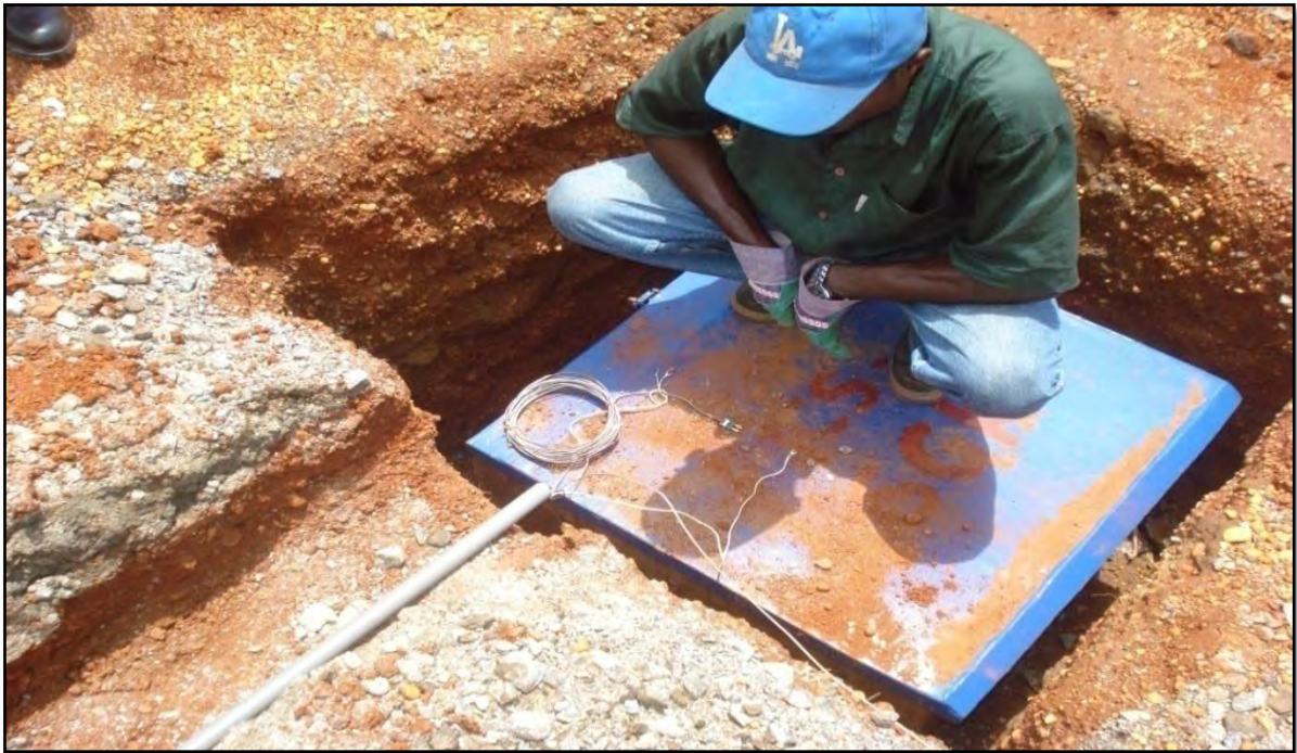
Figure 4.20 – View of Laterite Excavation
