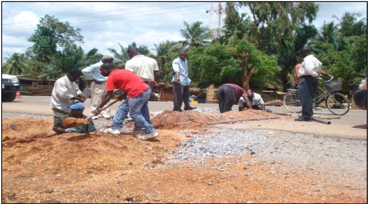
Figure 4.19 – Excavation of Site for Installation of Thermocouple and Soil Moisture Equipment
