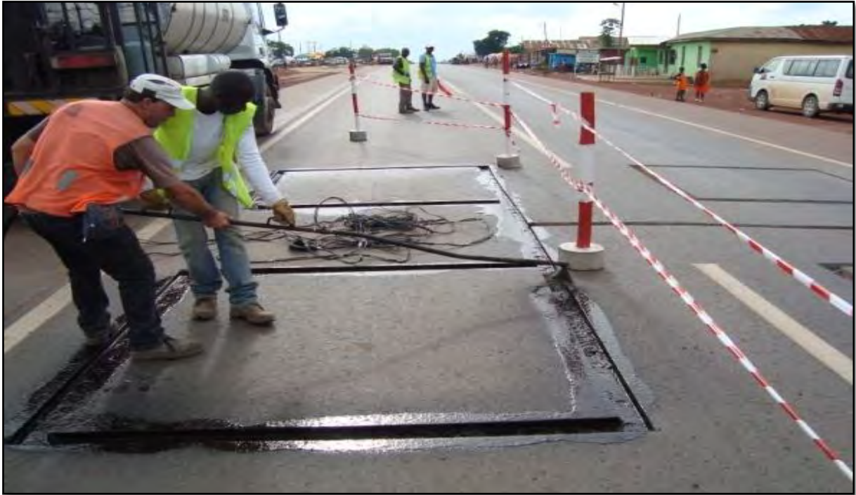
Figure 4.7 - Field Preparation for Installation of Induction Loop
