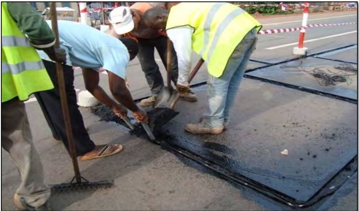
Figure 4.8 – Field Installation of Induction Loops
