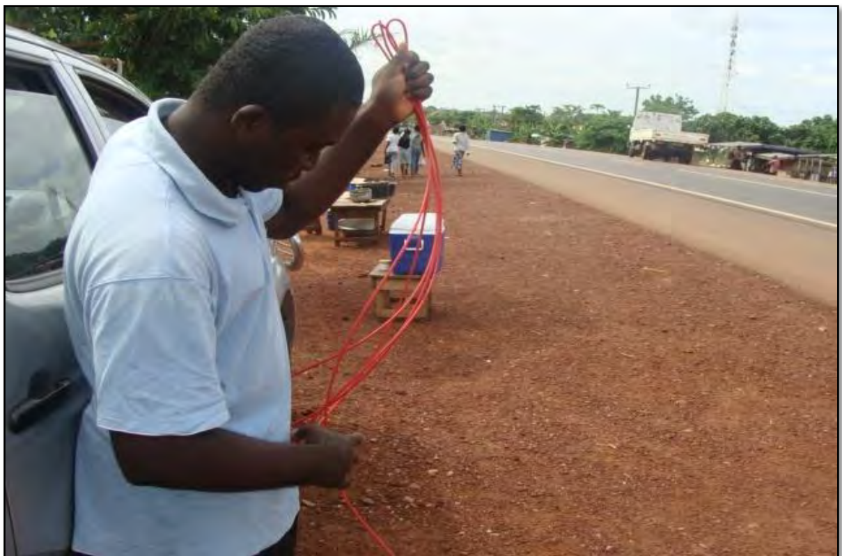
Figure 4.9 – Preparation of Induction Loops on Site
