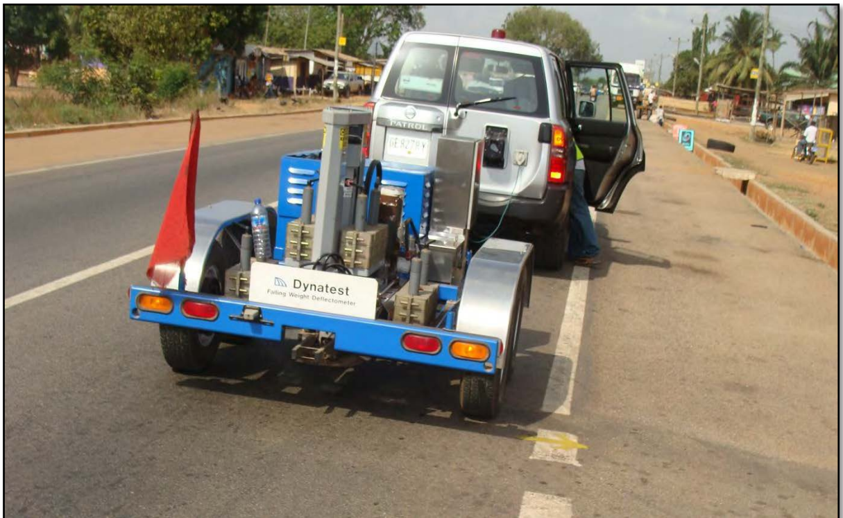
Figure 4.26 – The FWD Ready to Start Testing
