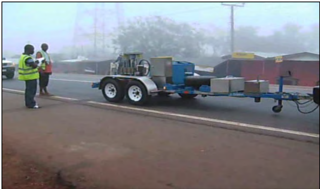
Figure 4.24 – Operation of FWD on Site
