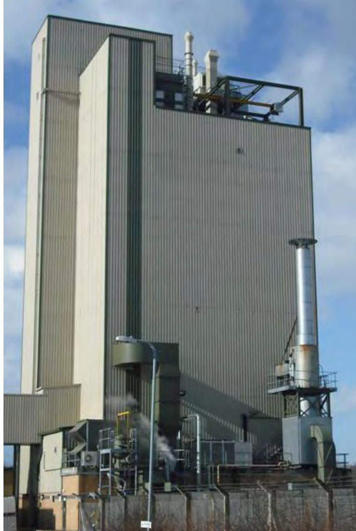
Figure 3.1: P&G Integrated Pilot Plant
