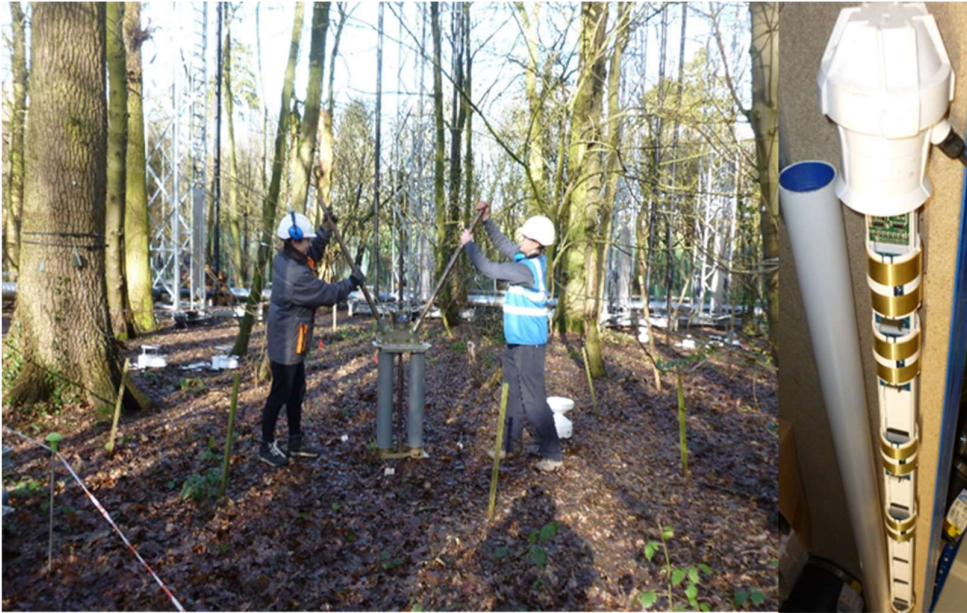
Figure 2- 4: installation of soil moisture profile probes
