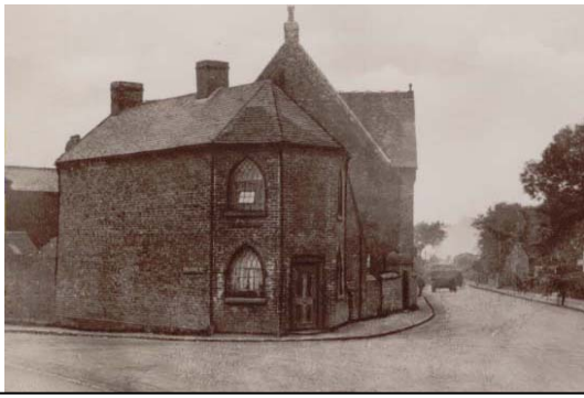
Quinton Toll House and Hagley Road Wesleyan Chapel
