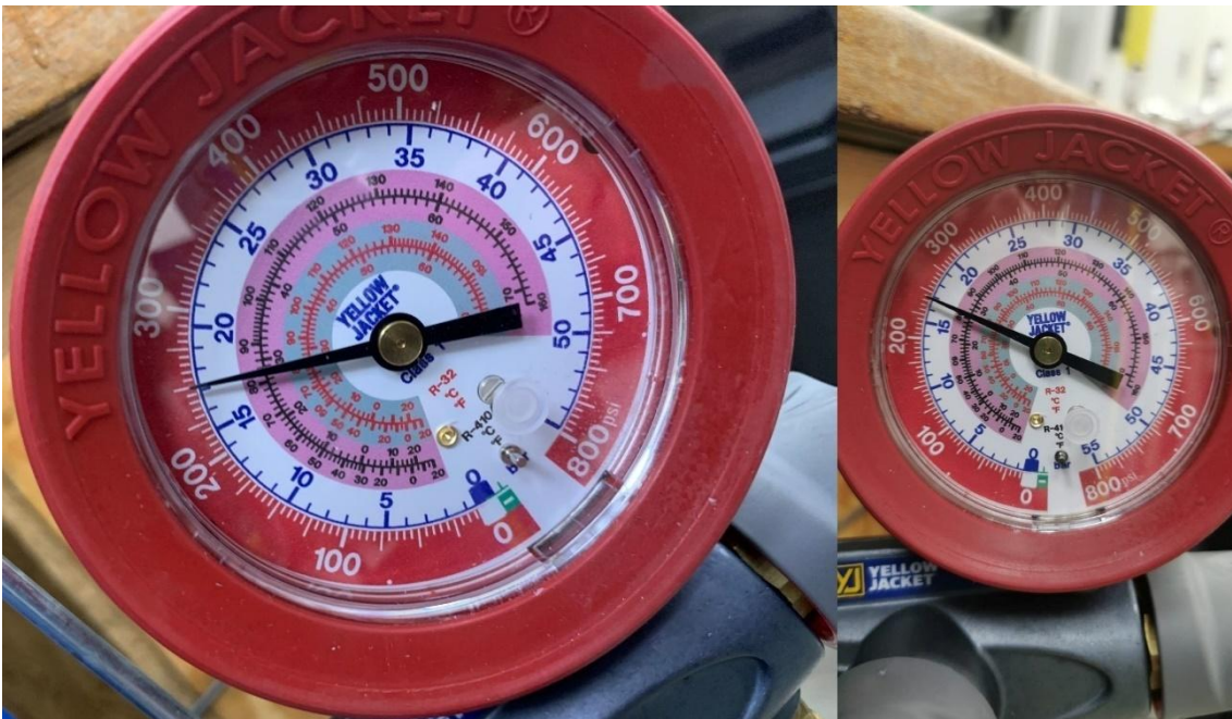
Figure 3.25: Tightness test reading on pressure gauge at 17 bars; 24 hours apart
