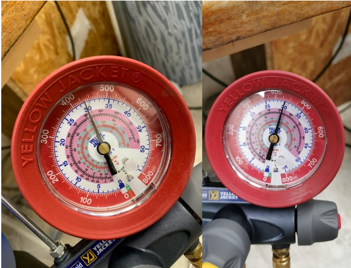
Figure 3.24: Strength test reading on pressure gauge at 30 bars; one hour apart
