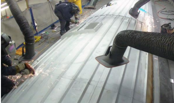
Figure 61 – Beginning of roof removal
