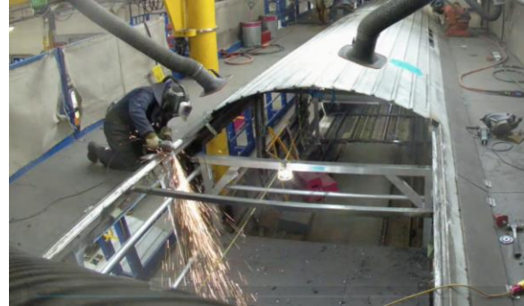
Figure 62 – End of roof removal
