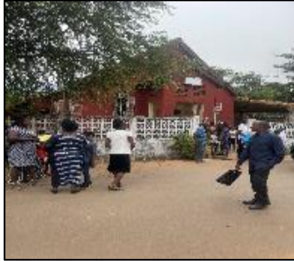
Figure 8: St. Luke's Parish Church
