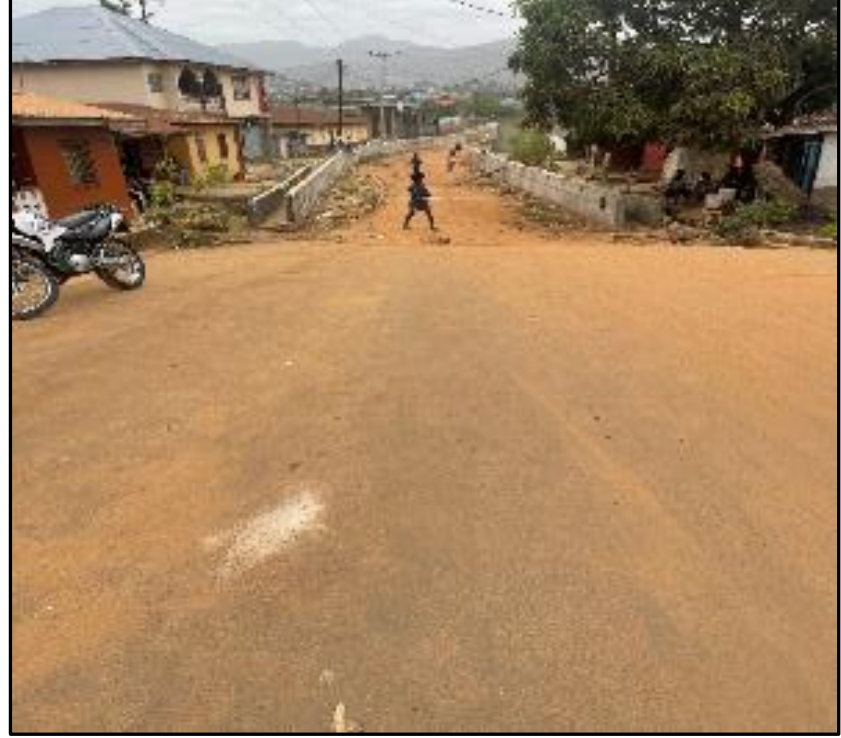
Figure 11: Freetown Road under construction
