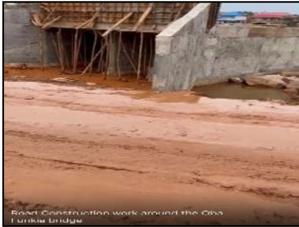
Figure 1: Construction Work at Oba Funkia Bridge
