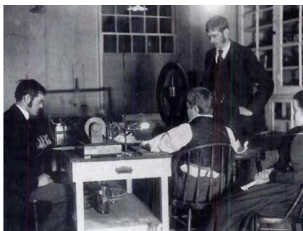
Figure 3.4: (Left) The Puluj's tube and induction coil that were used to take the first X-rays in the US at Dartmouth College. (Right) The moment the first X-ray was taken at Dartmouth College with (Left to Right) Edwin Frost, patient Eddie McCarthy, Gilman Frost, and Margaret Mead Frost [43].
