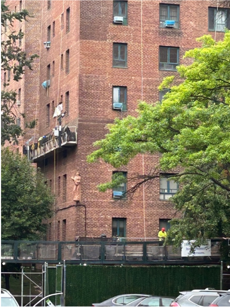
Figure 6.20: Masonry workers repointing and replacing brick close to one of the sculptures, June 2023.
