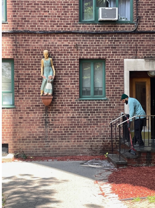
Figure 6.32: Parkchester buildings today are marked by the presence of air conditioners, green replacement windows and cable wiring all installed in the 1990s and 2000s during modernisation. Source: Author's photograph.
