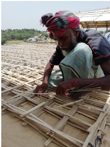
Rohingya elder weaving the bamboo connections in the camps of Cox's Bazar
