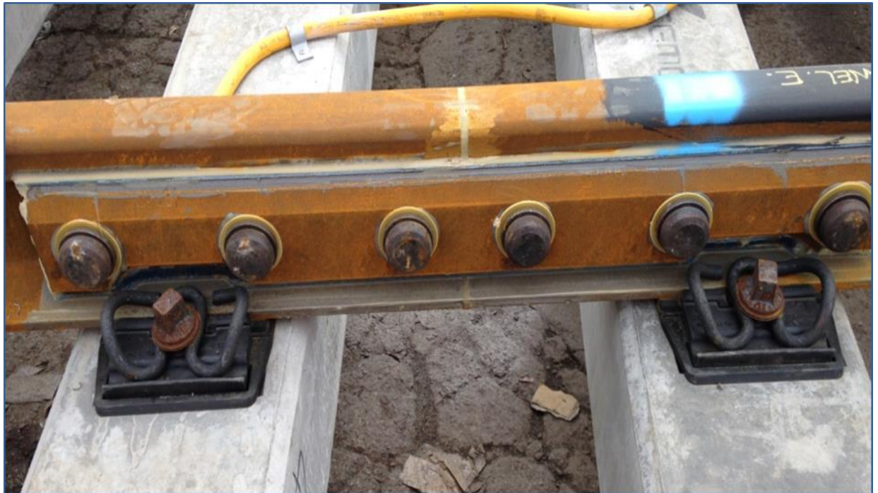
Figure 20: Direct Fixing based on Vossloh W21T System (Network Rail, 2017)
