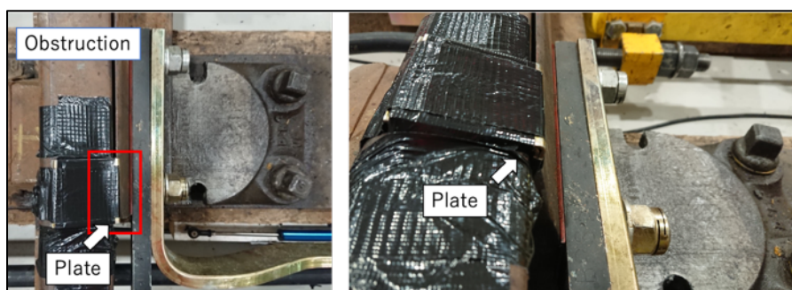
Figure 12. Obstructions between switch rail and stock rail
