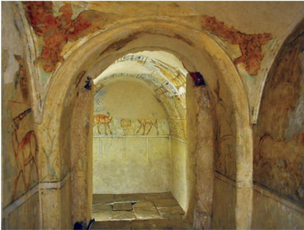
Figure 6b.16: The White Monastery crypt, looking into the barrel-vaulted burial chamber from the east. From Bolman et al. (2010: Fig. 5).
