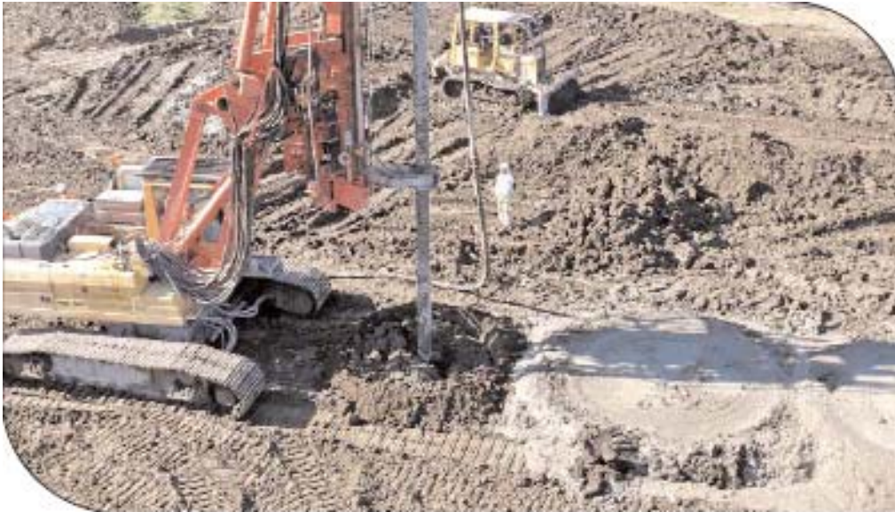
Figure 3:4: In-situ deep mixing of solidification columns (Wilk, 2005)
