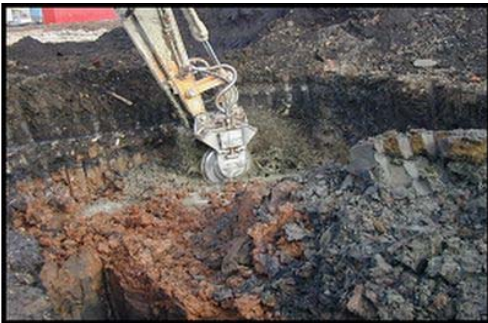
Figure 3:5: In-situ blender head in operation (Portland Cement Association, 2007)
