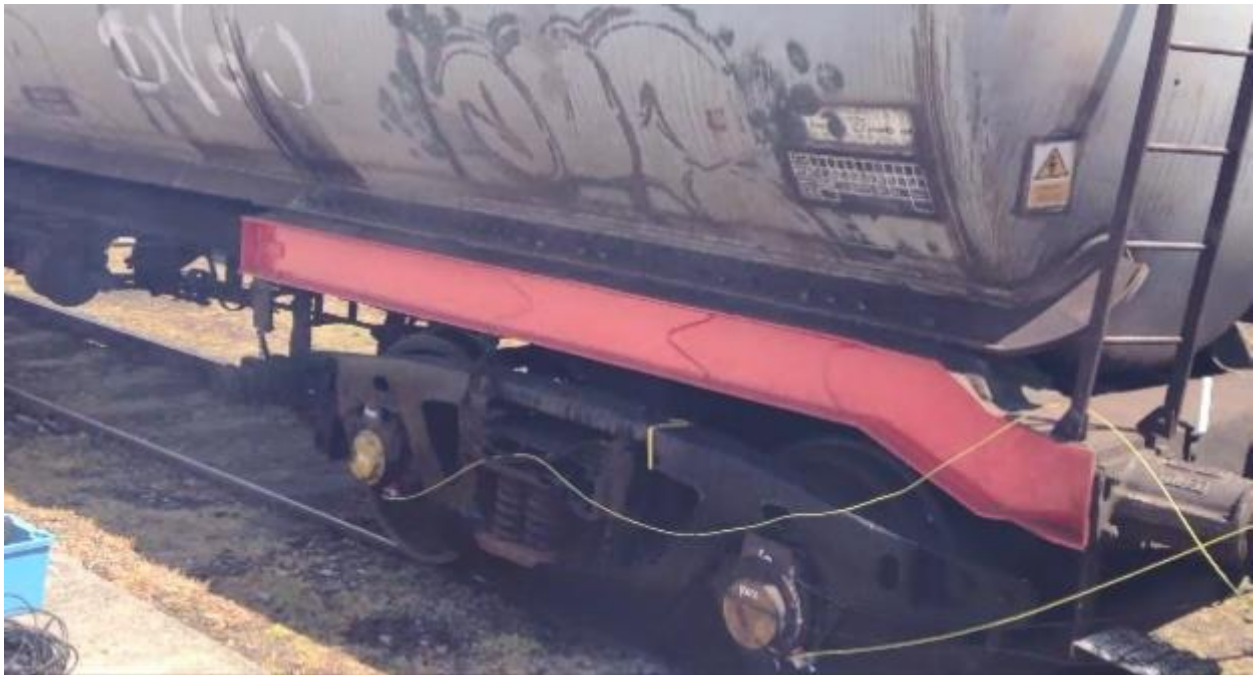
Figure 6-7: Onboard measurements of axle bearings with roller defects on the wagon tanker.
