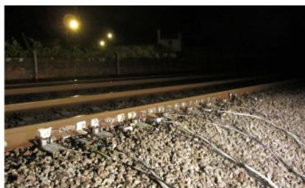
Figure 3-19: The actual site containing accelerometers and strain gauges (Meixedo et al., 2015).
