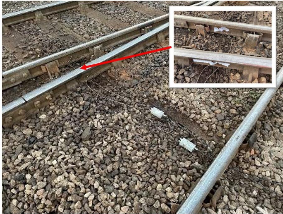
Figure 6-2: AE measurement system and the installation of two AE sensors
