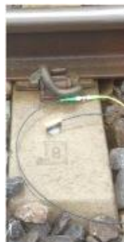
Figure 3-27: The accelerometer installed on the sleeper (Yüksel et al., 2018).
