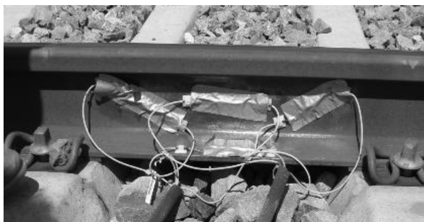
Figure 3-22: The actual condition of section 1 in Figure 20 (Filograno et al., 2013).
