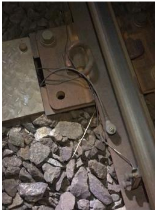
Figure 6-6: An AE sensor installed on one side of the rails.
