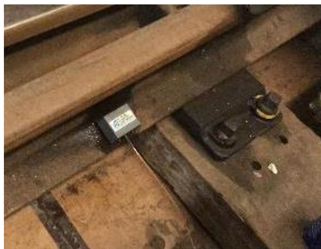
Figure 5-23: AE sensor installed by a magnetic hold-down.
