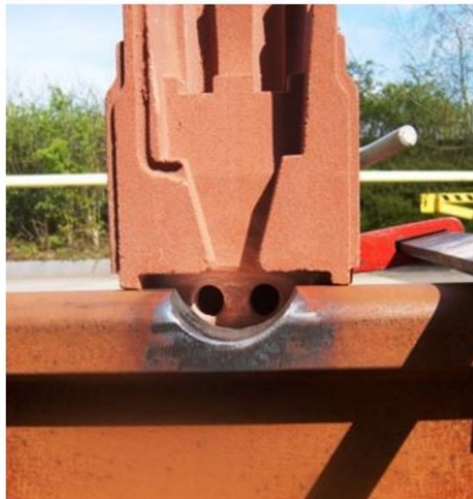
Figure 7.4 A mould onto the rail head after flame cutting [199].
