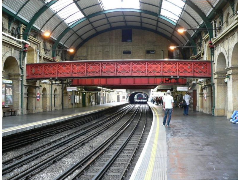
Figure 4.8 Paddington sub-surface station platform for the District and Circle lines (Source: McKenna, 2005, CC BY-SA 4.0)
