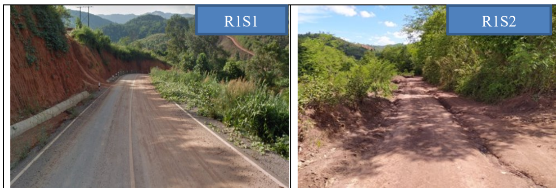
Figure 5-3 Road conditions for project 1
