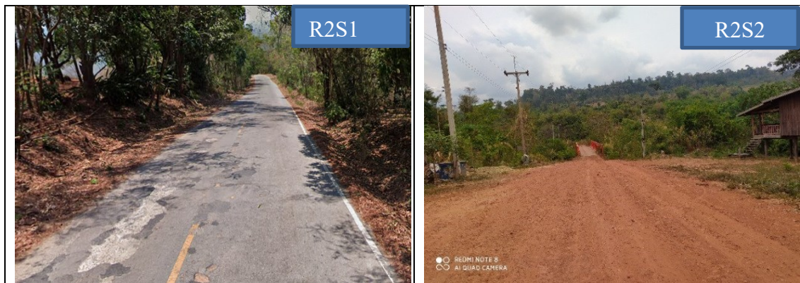
Figure 5-5 Road conditions for road project 2
