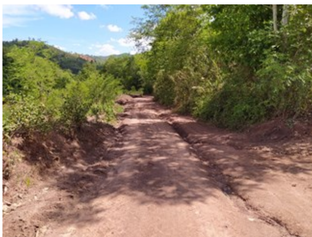
Figure A-1 very poor road condition
