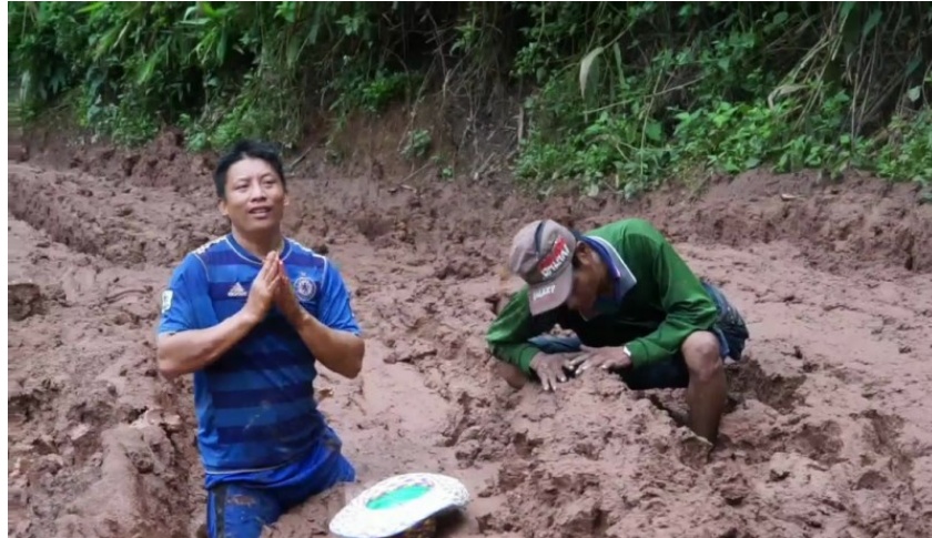
Figure 3-4. Condition of the road serving Sak Nga Village (source: Chiangmainews, 2019).
