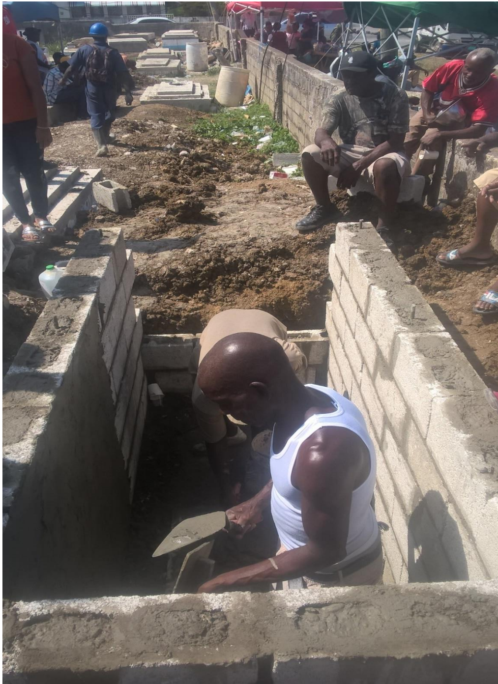
Fig 5.3 The sepulchre nearing completion. Source: Researcher's image.
