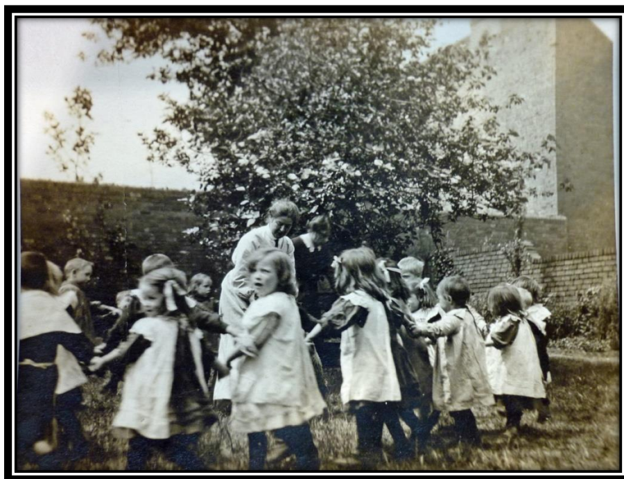
Figure 3.2: Summer Lane Kindergarten, The Settlement, Birmingham (c. 1907-1914) 49
