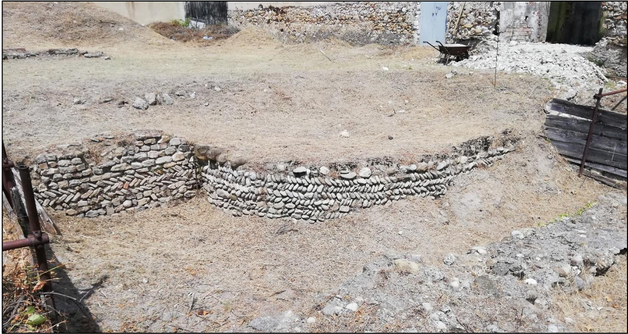
Figure 4.2) Albitimilium: The “Byzantine” wall, with the application of opus spicatum, near Porta Marina. (Source: Author)
