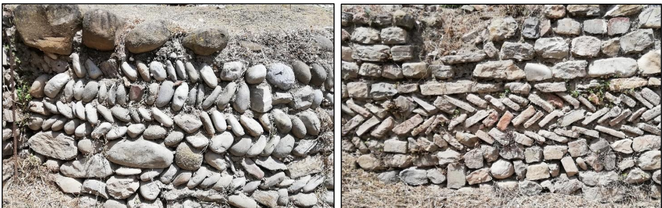
Figures 2.19, 2.20) Albintimilium: two different types of opus spicatum using pebbles and bricks from the area of Porta Marina. (Source: Autor)
