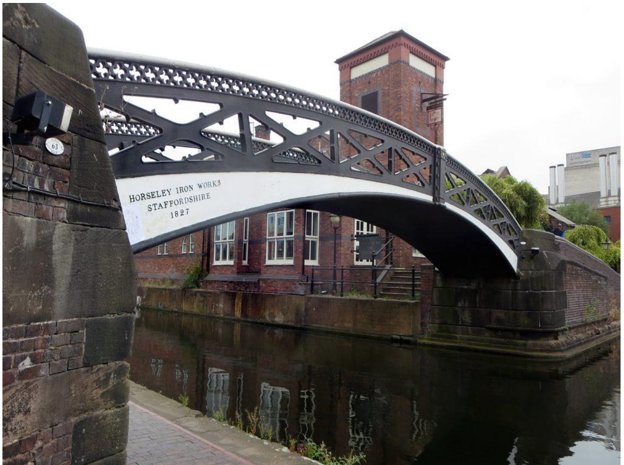
Figure 8: Cast-iron bridge (made by Horseley Iron Works) at the Old Turn canal junction, Birmingham 164
