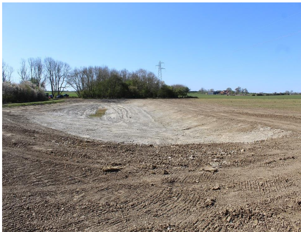
Figure 5.2 - Construction of the attenuation pond at Swaton as part of the NFM partnership project
