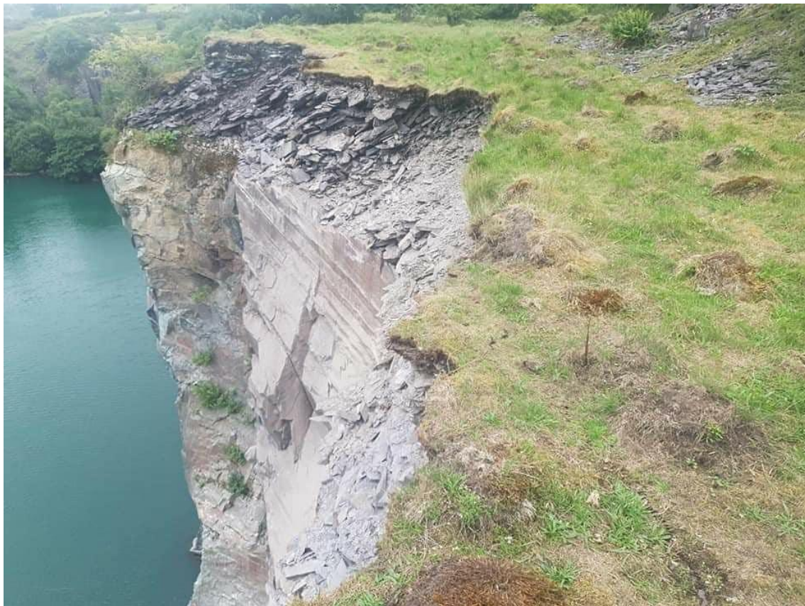
Figure 6-2 View of the backscarp of the failure (courtesy of Nigel Spires).
