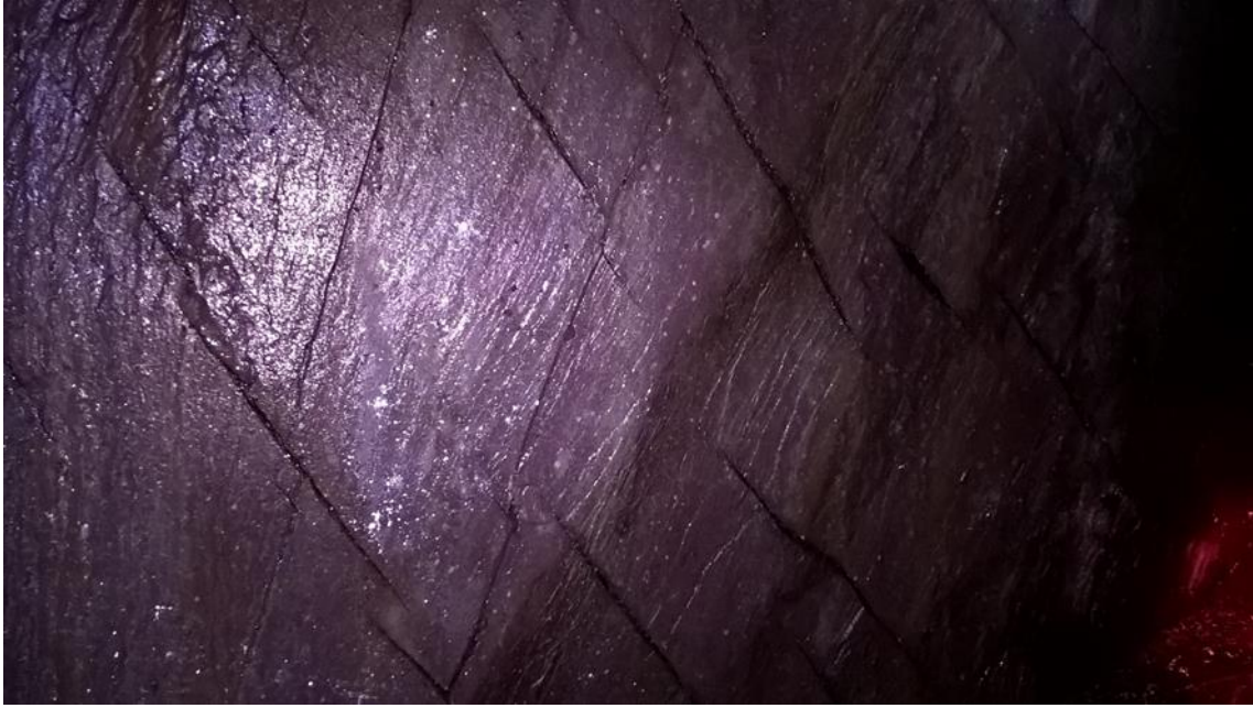
Figure 3-3 Apparently conjugate joints in an adit within the Llanberis Slates.
