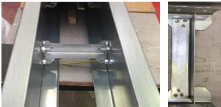
Figure 3.3 Typical angle strut and connection of strut and purlins.
