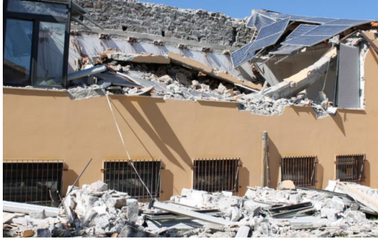
a) Roof collapse with solar panels of a library building in Italy for gravity loads, in 2015
