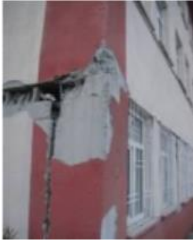
a) Beam-column joint failure due to low shear strength of beams, inadequate shear capacity of columns and poor concrete quality (Ilki et al. , 2012)
