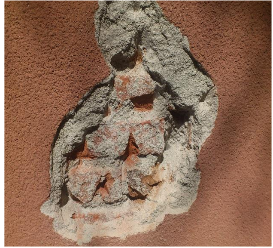
b) The concrete surface removing for determining structural material
