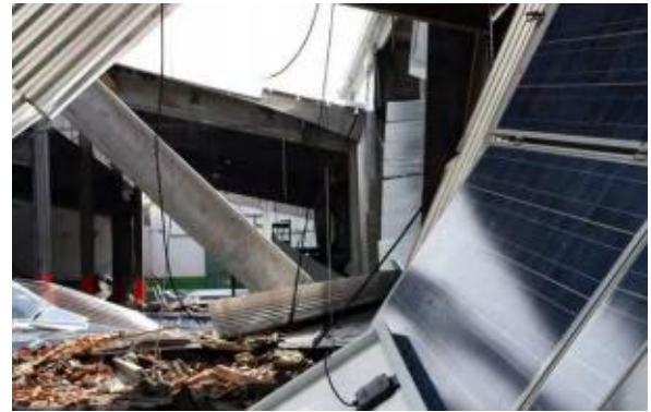
d) The collapse of an industrial warehouse renovated with photovoltaic panels in Italy after the Emilia earthquake in 2012
