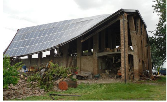
b) Roof collapse with solar panels of a building in Italy after Emilia earthquake in 2012
