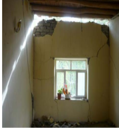
b) Cracks on non-load-bearing wall (in the middle) due to insufficient connection in roof-floor joints and out-of-plan motion caused by height and thickness of the wall (Güney, Kuruşcu and Arun, 2016)
