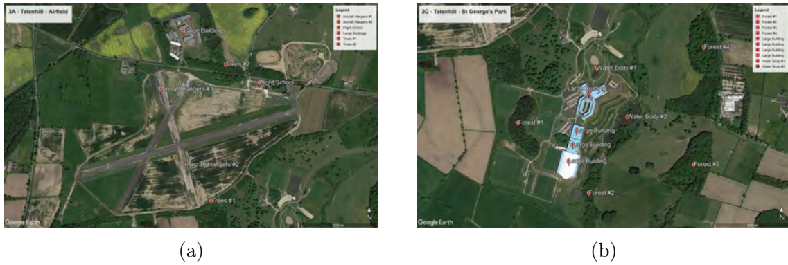
Figure A.4: Aerial images of sub-regions of the tatenhill target area showing a close-up of (a) the airfield runways, and (b) the buildings within St George's Park
