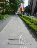
Figure 6-55 Different design of the concrete drain covers replacing the steel grating
