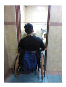
Figure 6-21 Inaccessible toilet door opening for wheelchair
