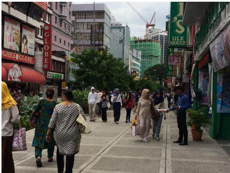
Figure 24 Completed JTAR walkway upgrading to a barrier free design that begun in 2012. Source: Author, 2017.
