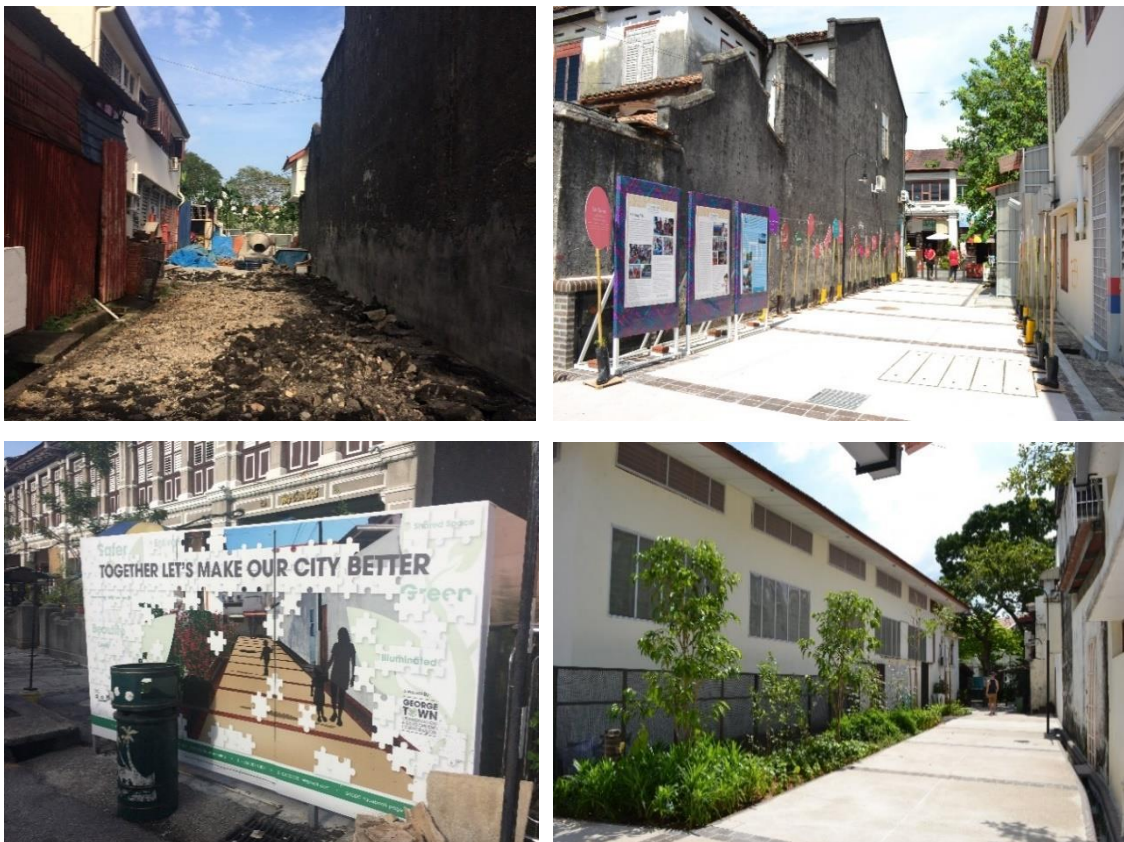
Figure 27 Several improvements on laneways connecting to Armenian Park during fieldwork. Source: Author, 2017.
