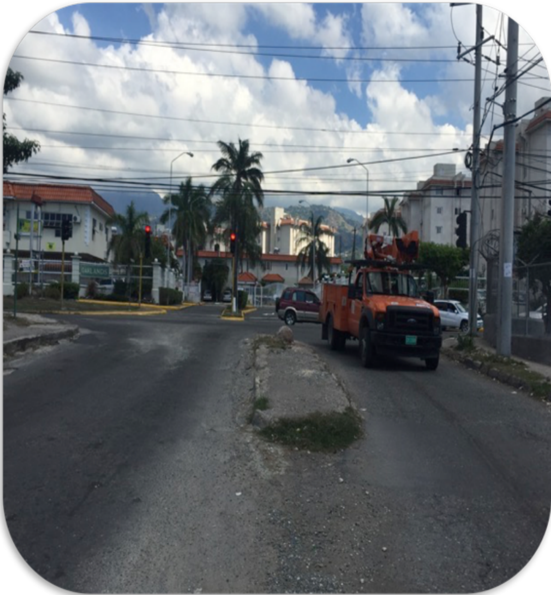
Figure C.1 Image showing condition of median
