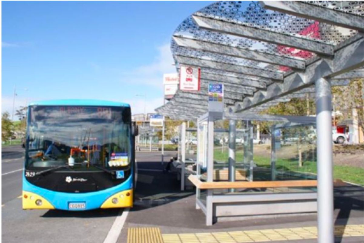
Figure 2.10 Bus border stop and bus shelter facilities provided for public transport pedestrian users. Modified by Uter (2018) and obtained from NZTA (2014)
